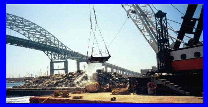
Material is inspected prior to use at the reef. Rebar, asphalt, and paint are removed or trimmed from materials.
