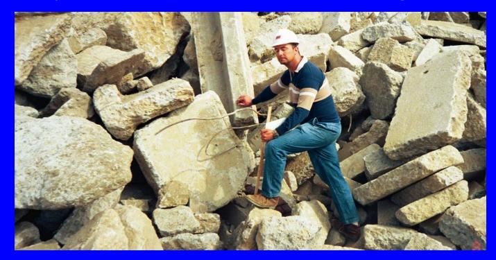
• Material is sorted prior to use at the reef to meet the size specifications for reef design.
