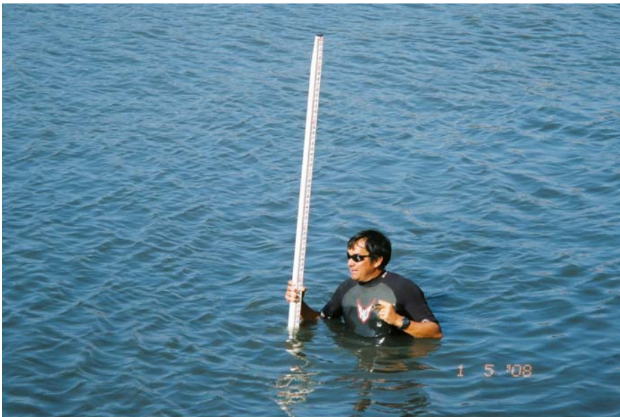
Photographs showing Joe Ellis checking the excavated bottom elevation.
